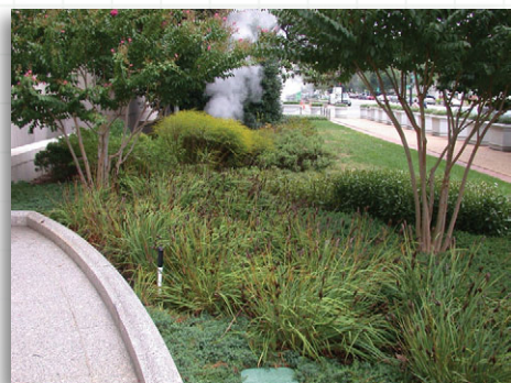
A bioretention cell, also called a rain garden, is one of the LID practices being demonstrated at EPA Headquarters.
