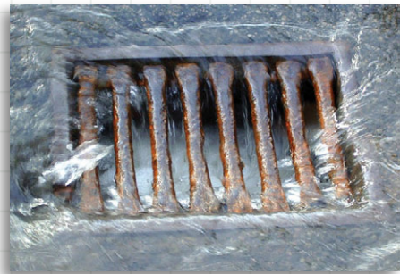
Stormwater runoff from roads, parking lots, and other impervious surfaces flows into storm drains, which lead to nearby waterbodies.
