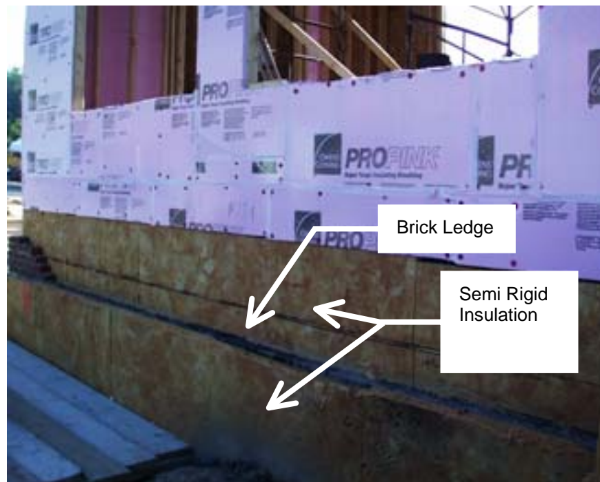
Figure 4. Insulation of foundations below grade at Estate Homes showing brick ledge
