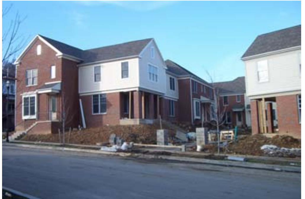
Figure 3. Building 1 of the Rental Town Homes at Summerset nearing completion
